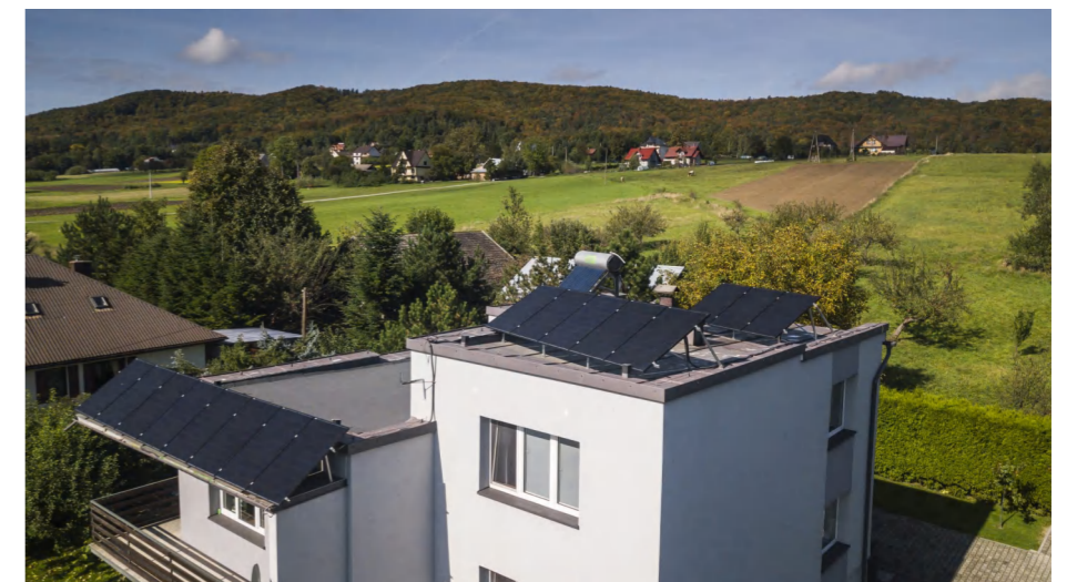
Netherlands System Capacity: 10kW
