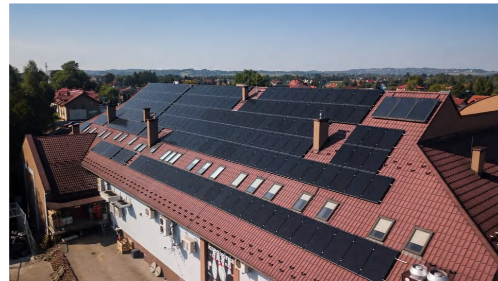
Sweden System Capacity: 30kW
